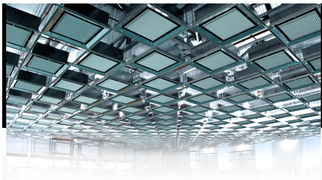
Figure 1. Schematic illustration of FFU (fan filter unit) installation in a semiconductor cleanroom.
