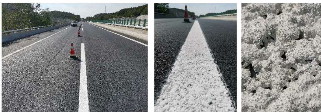
Figure 15. Test section after marking application.
