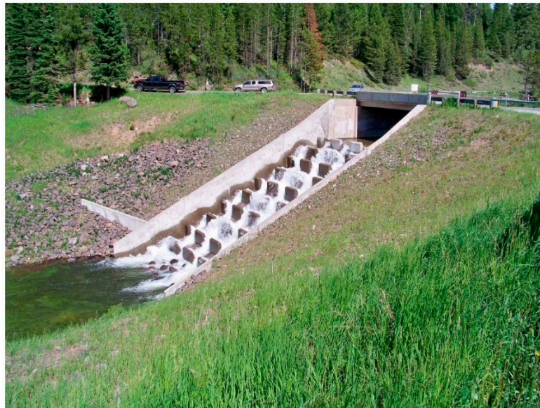
Figure 1. Example baffled chute spillway in Bozeman, Montana USA (photo from C. Brown).
