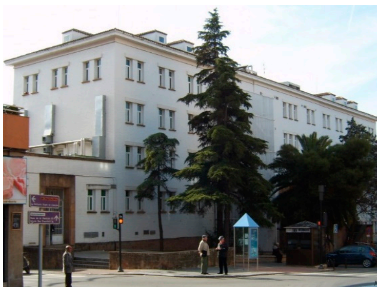
Figure 1. General view of the Virgen de Linarejos Health Center.
