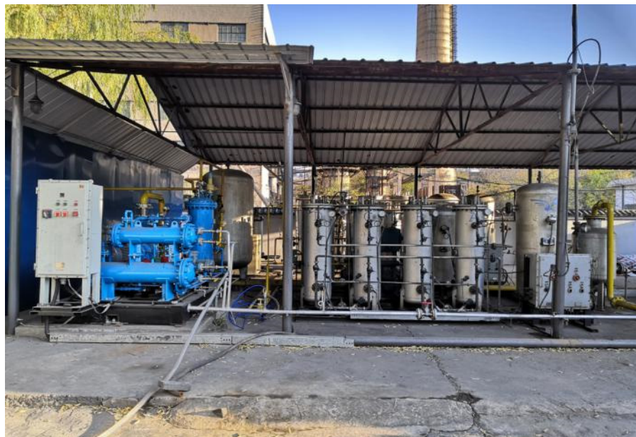
Figure 6. Four-tower coalbed methane separation device using PSA.
