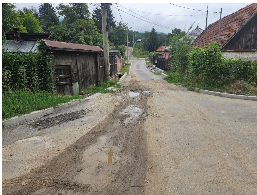
Figure 12. Area where mine gas drainage works were carried out.
