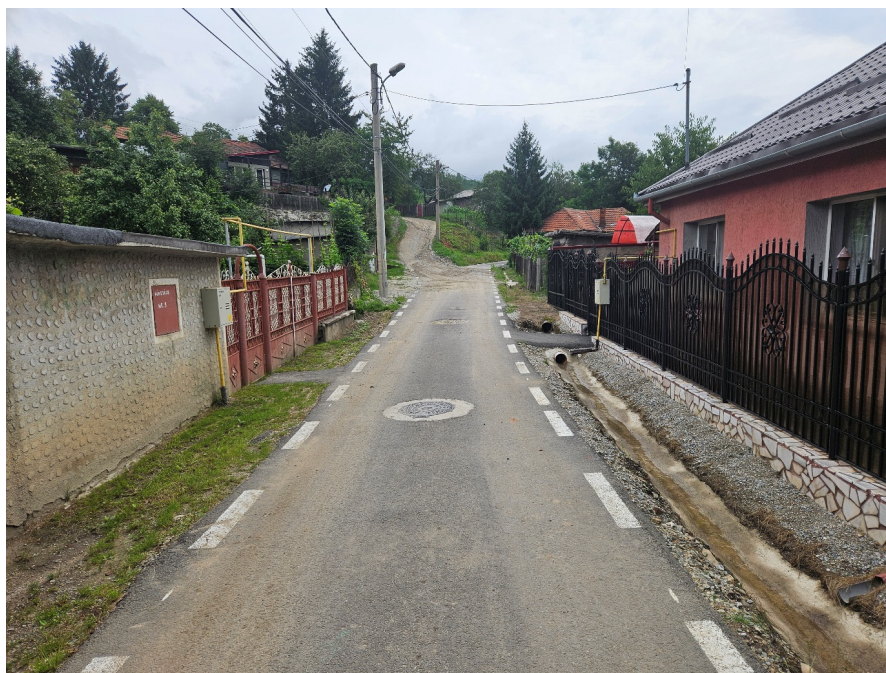
Figure 13. Rehabilitated area and pipeline back in operation.
