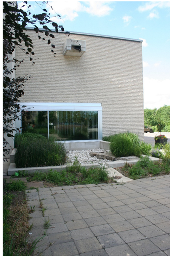
Figure 13. A view of the roof scupper and wetland (Credit: Roberto Chiotti).
