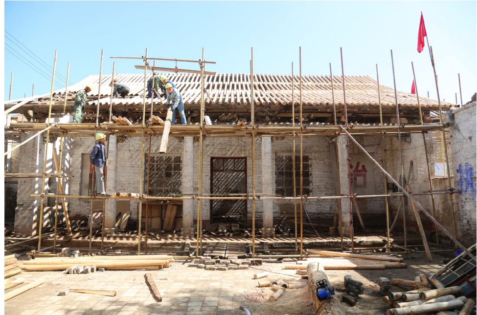
Figure 4. Guozhuang Lord Guan Temple under restoration.
