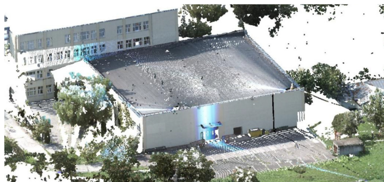
Figure 9. The final TLS point cloud resulted after georeferencing four individual point clouds.
