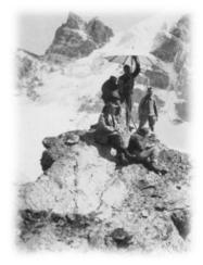
**Figure 4.** A terrestrial phototheodolite station in Switzerland, although post-1925, cadastral surveys were almost exclusively completed using aerial survey (adapted from [53]).
