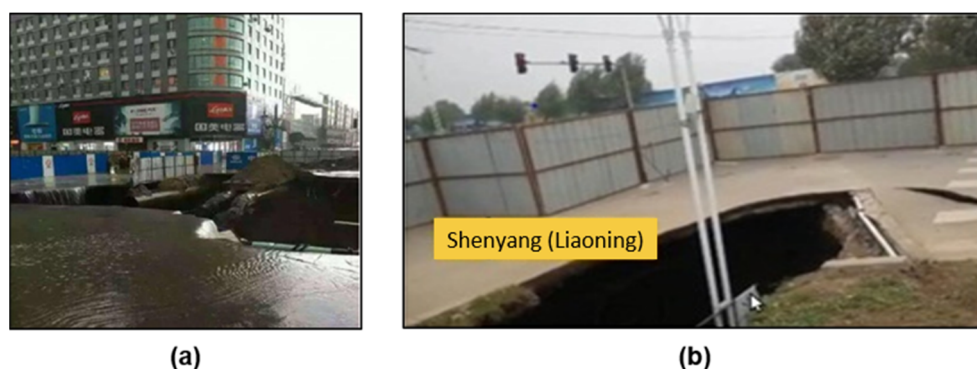
Figure 14. Images of reported collapse events along subway lines: (a) collapse at the intersection of line 1 and line 9; (b) collapse at Caozhong station (marked by red triangle in Figure 13a), line 9.
