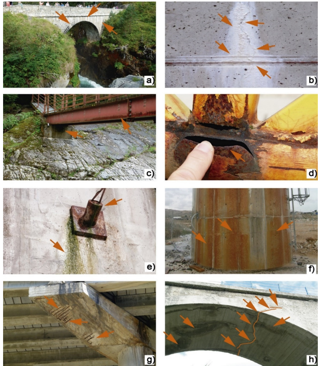
Figure 3. Some common damages that can affect bridges: (a) efflorescences on a masonry bridge in Cauterets, France; (b) efflorescences and crack in a reinforced concrete wall; (c) lichen growth in abutment and corrosion of a steel bridge beam in Lanuza, Spain; (d) crack and corrosion in steel truss handrail in Alcoy, Spain; (e) lichen growth caused by excessive humidity and corrosion in cable anchor plate in abutment in Benidorm, Spain; (f) rust stains in a surge chamber; (g) concrete spalling due to corrosion of steel reinforcement in a bridge in Petrer, Spain; (h) transverse cracks on reinforced concrete arch of bridge in Alcoy, Spain.
