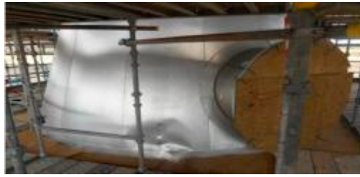
Damage to brine concentrator—post-impact.
