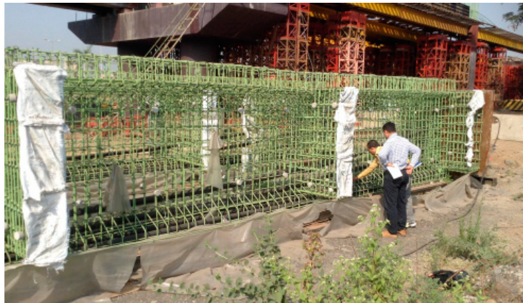
Figure 5. Sensors on reinforcement cage.
