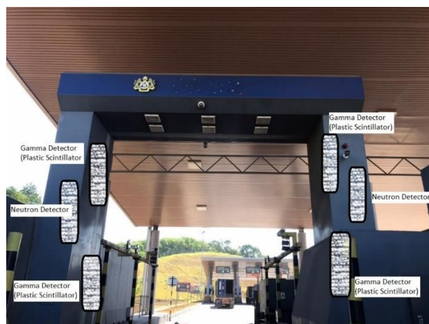
Figure 3. A radiation portal monitor at customs and immigration check point Bukit Kayu Hitam, Kedah, Malaysia.
