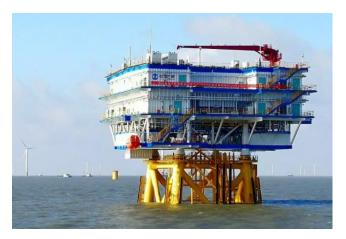
Figure 15. Offshore booster station.
