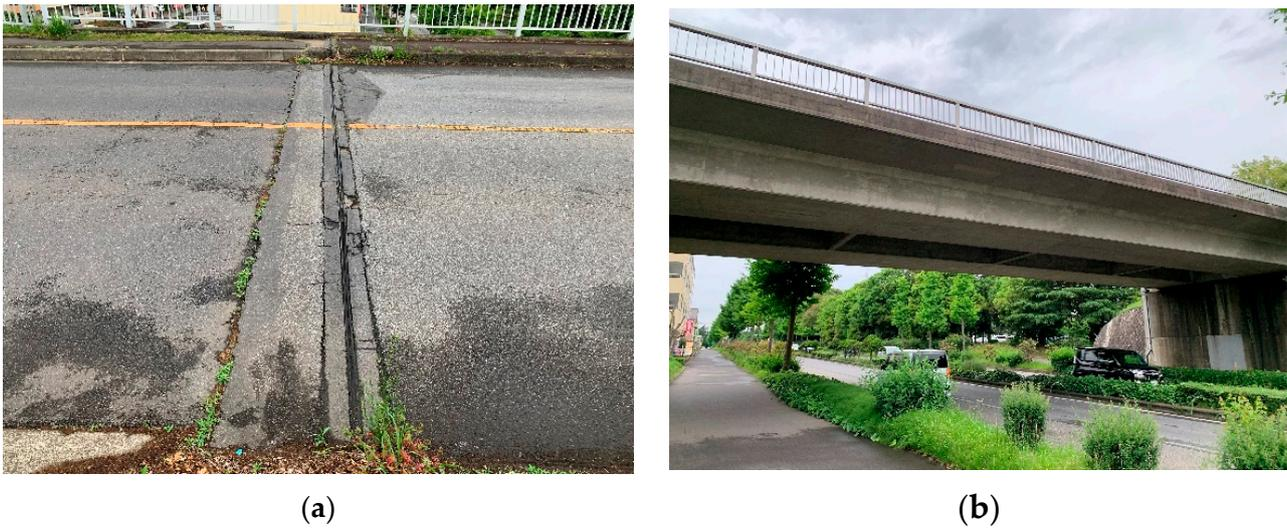
**Figure 5.** Photo of Bridge A: (a) rubber joints for bridges; (b) general view.
