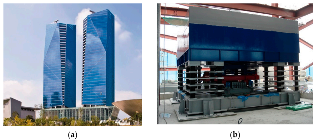
Figure 1. Benchmark structure: (a) Overview of the Posco E&C Tower in Songdo, South Korea; (b) 160 ton tuned mass damper.
