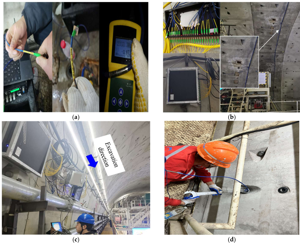
Figure 6. On-site monitoring system installation of Internet of Things: (a) sensor initial value reading; (b) data aggregation and transmission; (c) real-time data check; (d) installation of bolt stress gauge.
