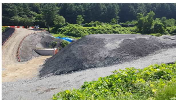
Figure 1. Construction of the model slope.
