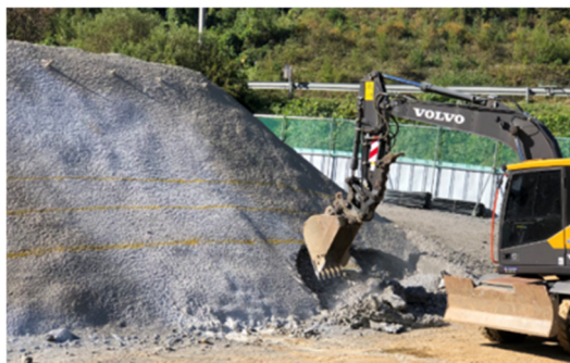
Figure 10. Excavator excavating slope.
