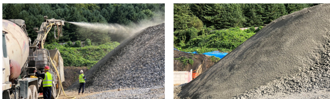
Figure 9. Shotcrete operation process and completion scene.
