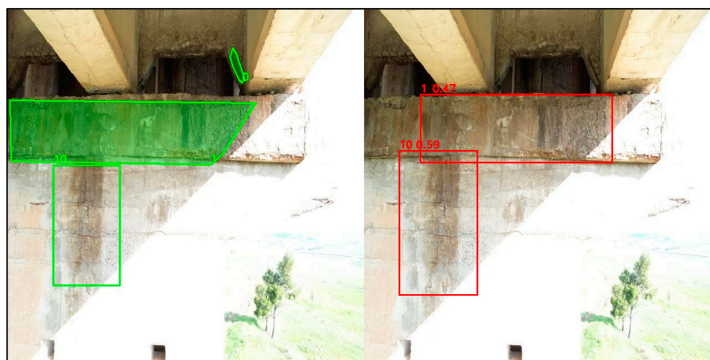
Figure 8. GT and YOLO prediction comparison on an image from bridge #7.
