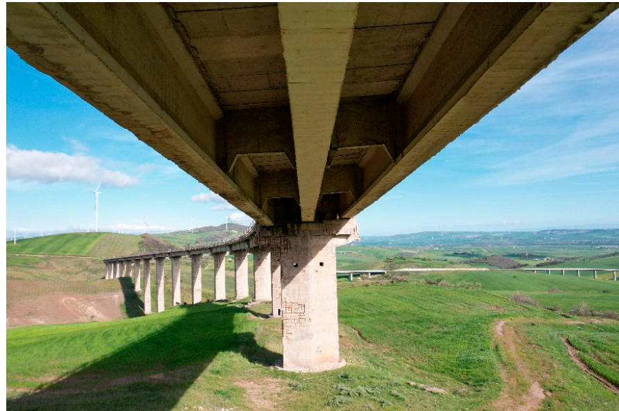
Figure 1. Typical panoramic inspection image.
