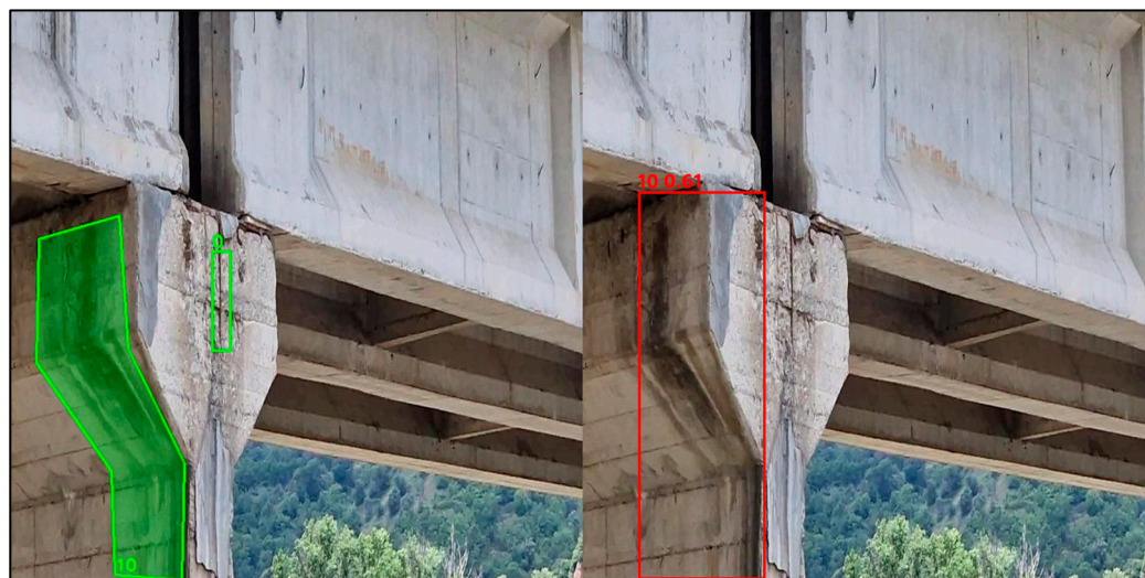
Figure 9. GT and YOLO prediction comparison on an image from bridge #8.
