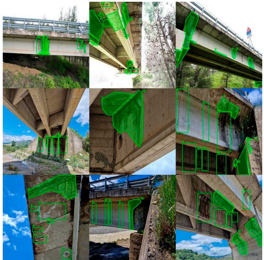
Figure 5. Example of image annotations through polygons and rectangles (pictures belonging to the training set). The numbers correspond to the classes in Table 4.
