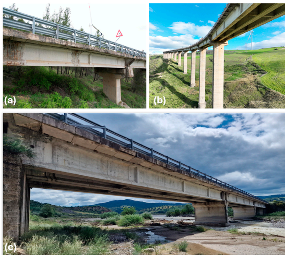
Figure 4. Views of some of the examined bridges: (a) bridge#1, (b) bridge #7 and (c) bridge #8.
