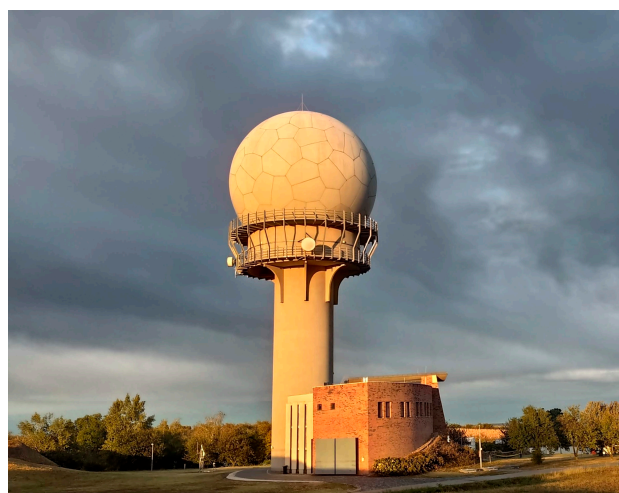
Figure 2. RAT-31DL 3D radar tower.
