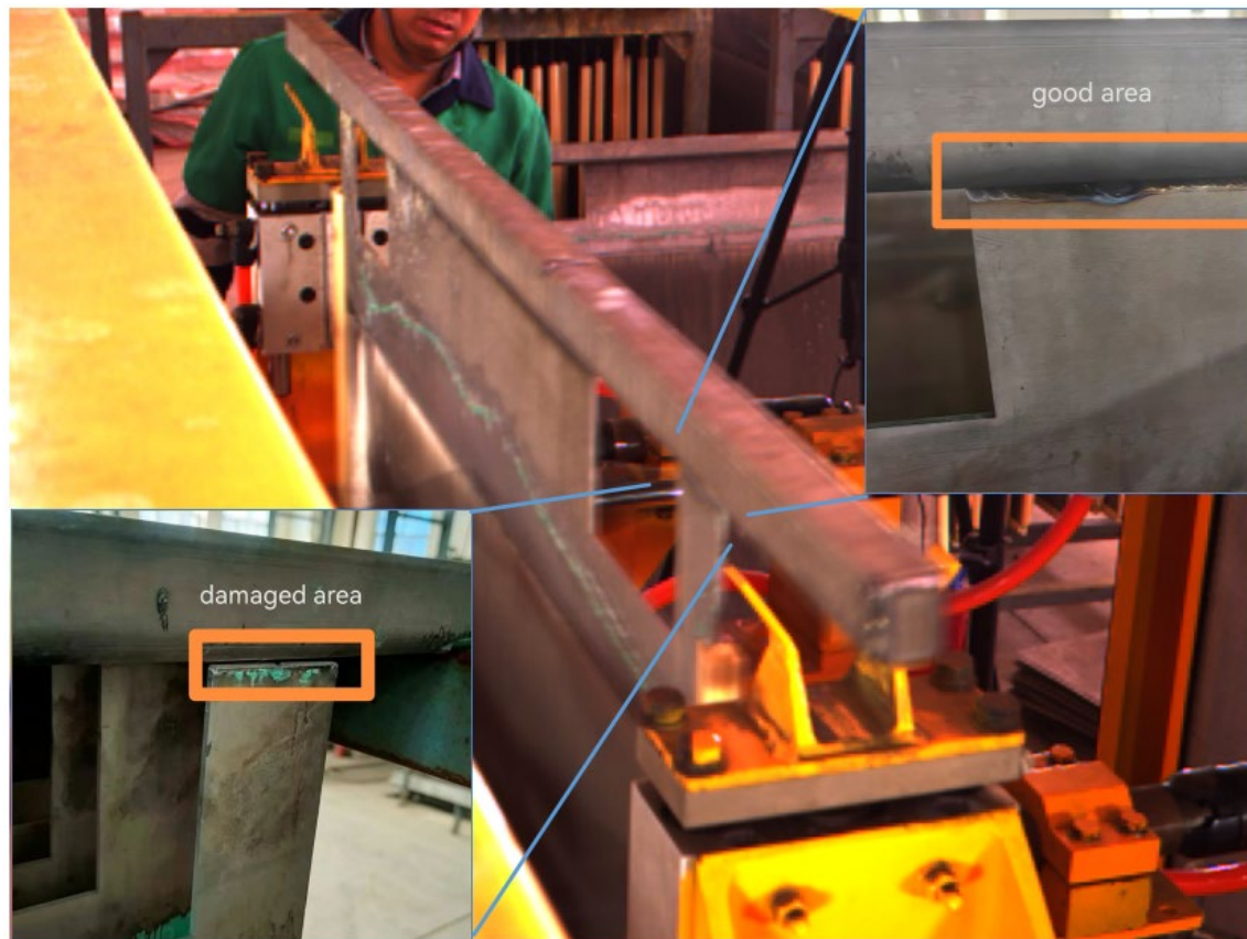
Figure 10. Comparison of visible titanium starter-plate connection damage before and after tamping.
