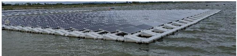
**Figure 4.** Illustration of the typical pure-float FPV system which is considered in this study.
