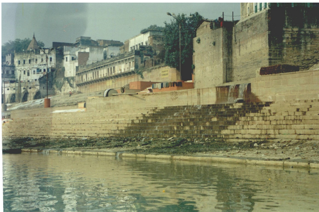
Figure 3. Raw sewage flows into the Ganges in Varanasi.
