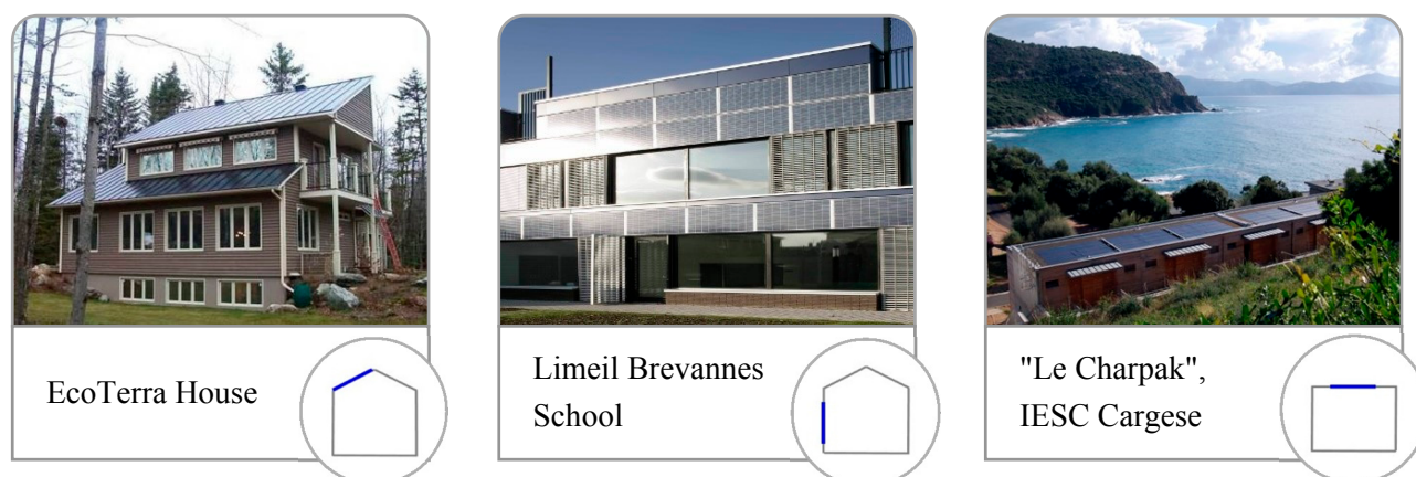
Figure 4. Categorization of PV installation method: integrated type [33].
