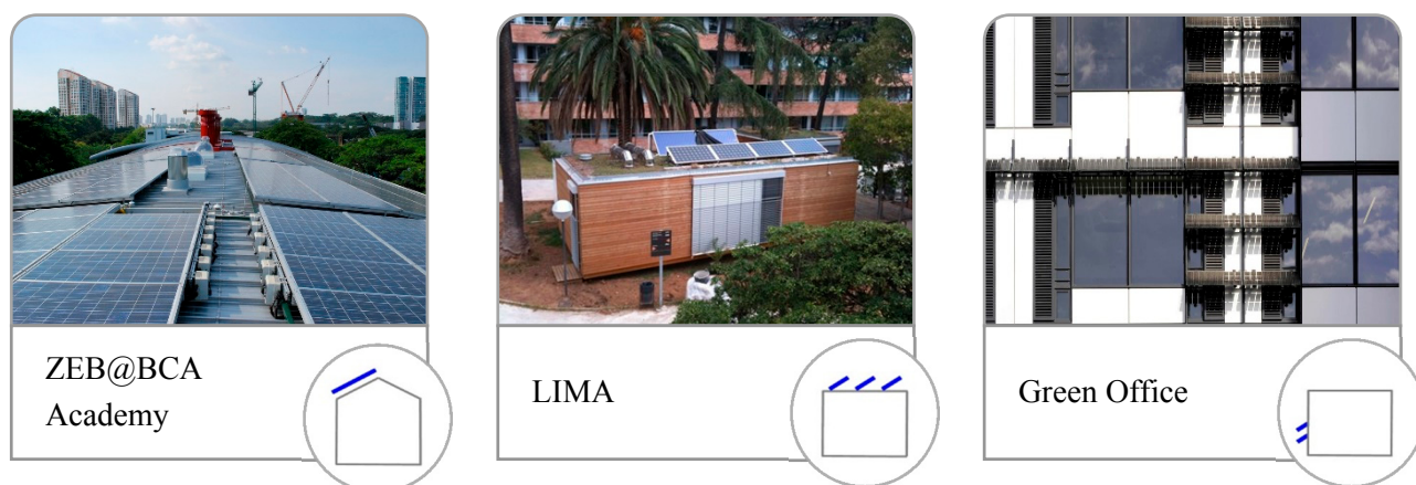
Figure 5. Categorization of PV installation method: non-integrated type [33].
