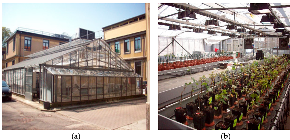
Figure 1. (a) Greenhouse external structure; and (b) disposition of counters, pots, lighting and cooling systems.
