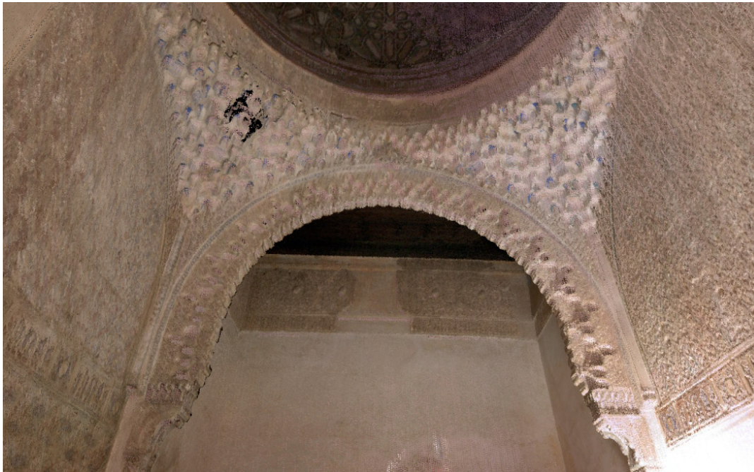
Figure 16. Pendentives in the Sala de la Barca (point cloud).
