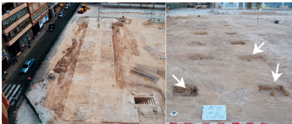
Figure 3. (left) View of the entire shelter from a neighbouring building in the aftermath of the demolition of the buildings that were built on top of it in the post-war years. (right) View showing the inlaid vents in the concrete slab.
