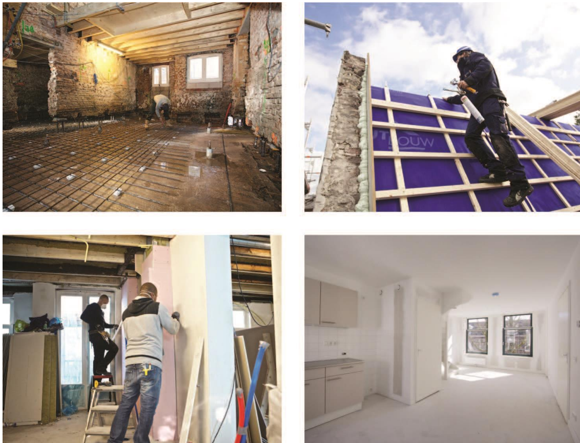
Figure 3. The expensive integral box-in-box-renovation of Czaar Peterbuurt block N46. Top left: Renovation of load bearing walls and foundations. Top right: Roof is replaced. Bottom left: Walls are covered. Bottom right: New apartment with a new floorplan. Photos by Mercuur Bouw.
