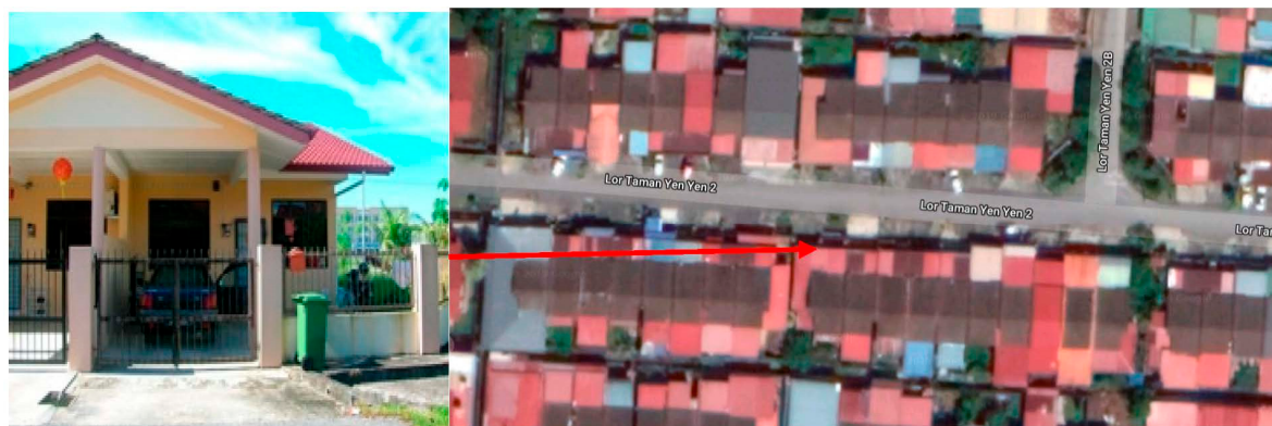
Figure 2. Case study building (left) and location of the case study house (right).
