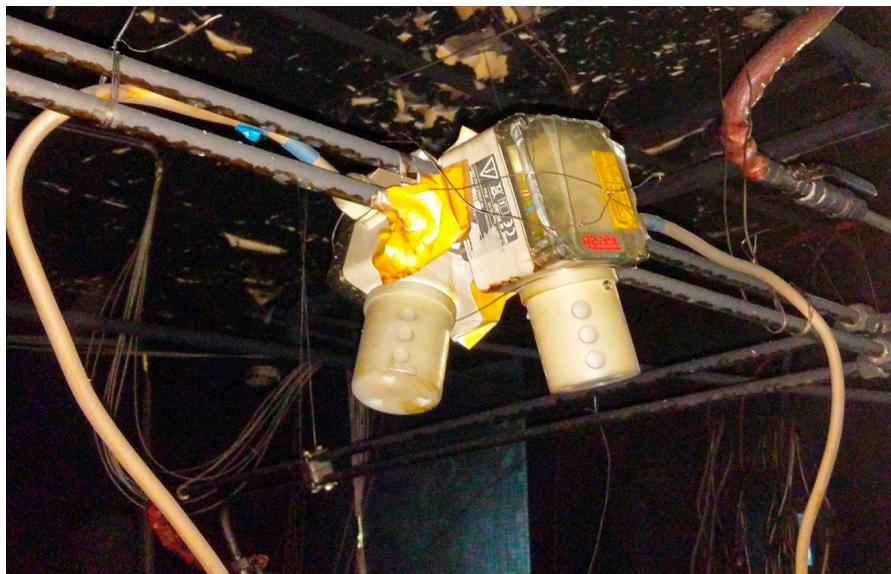
Figure 6. A view of oxygen and carbon monoxide sensors.
