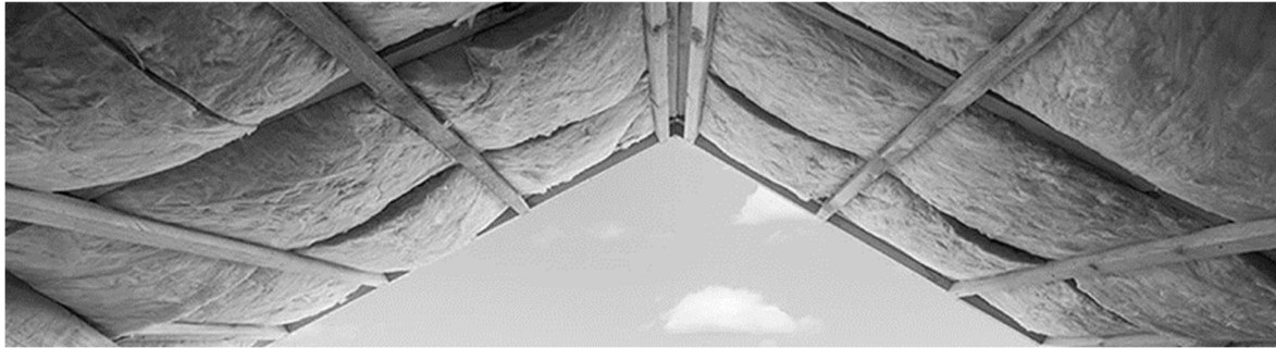
Figure 5. Example of sheep wool insulations on roof [41].
