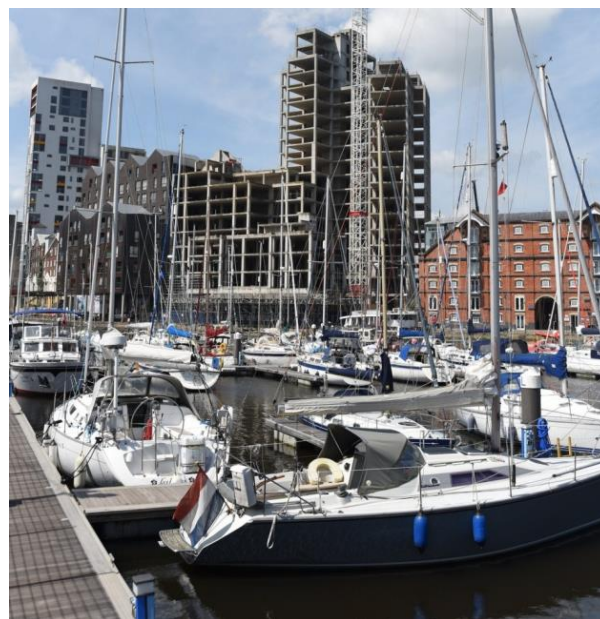
Figure 4. A large building left unfinished since 2010 on Ipswich’s Regatta Quay, along the Orwell river. Relying on limited uses and basing the project’s success on the premise of high-return renders it vulnerable to boom-and-bust economic cycles (image credits: Angela Sharpe/Ipswich Star, used by permission).
