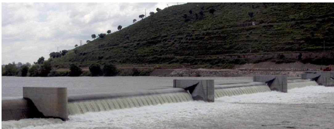
Figure 2. Abrantes' inflatable weir-dam (image: TPF Consultores, used by permission).
