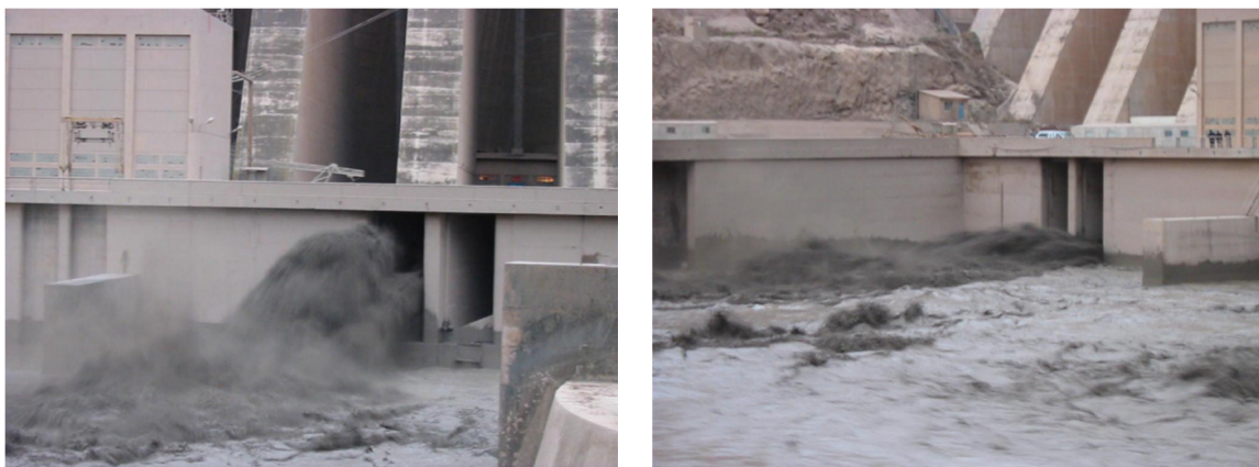
Figure 9. Sediment shock load released from Manjil Dam, Iran, during the storage restoration process in 1982–1983, which caused ecological disaster and a massive extinction of aquatic life downstream.
