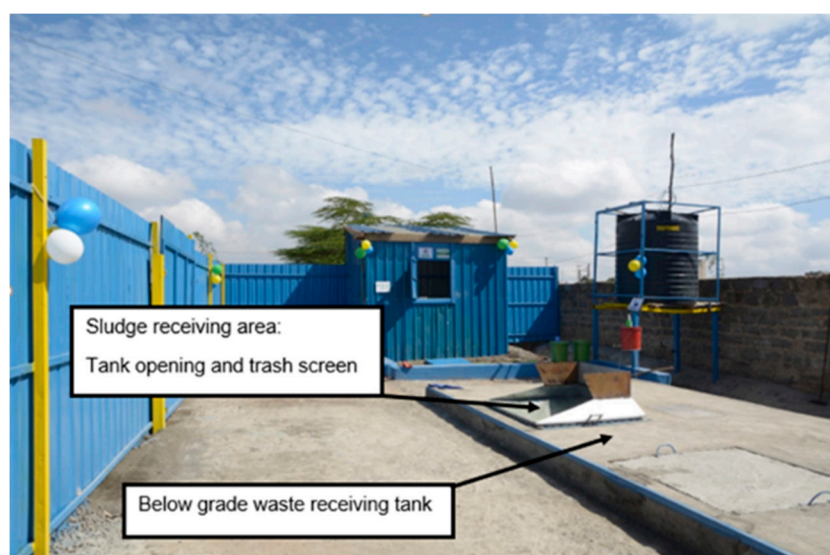
Figure 1. The Mtaa Fresh site contains a below grade tank in which pit latrine sludge is received from manual pit emptiers in Mukuru Kwa Njenga in Nairobi, Kenya. FS is delivered to the site in barrels. The contents of the barrels are tipped through a trash screen and into the tank. Photo Credit: Sanergy.
