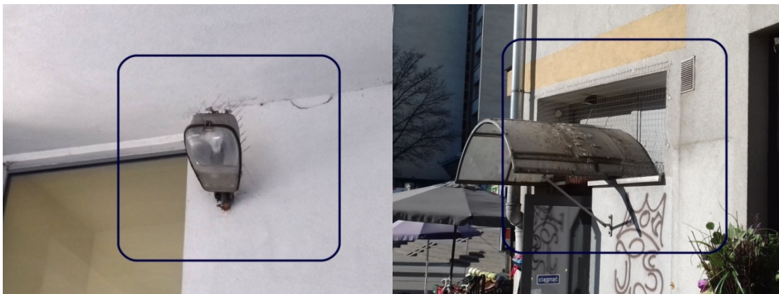
Figure 1. Bird spikes protecting urban infrastructure: lighting and roofing. Photographs by: K. Król.
