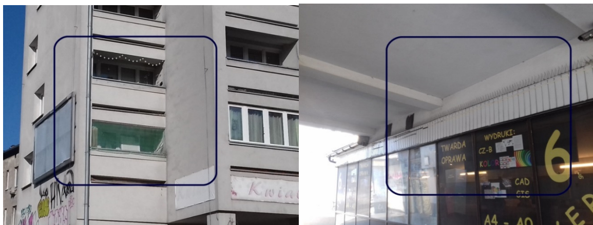
Figure 2. Bird spikes protecting urban infrastructure: balconies and cornices. Photographs by: K. Król.
