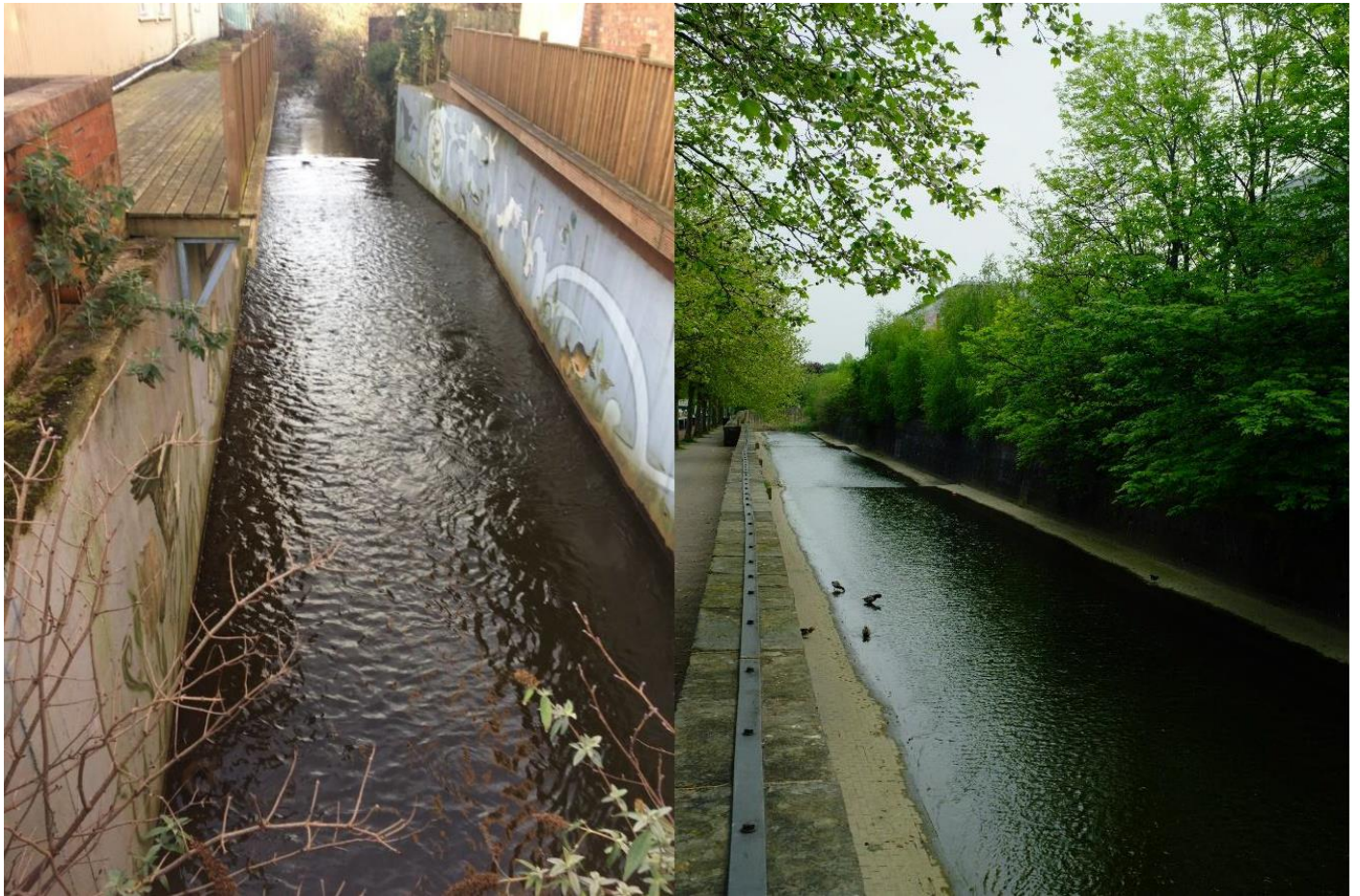
Figure 7. Examples of heavy river channel modification in Sheffield. Photograph: DCRT 2021.
