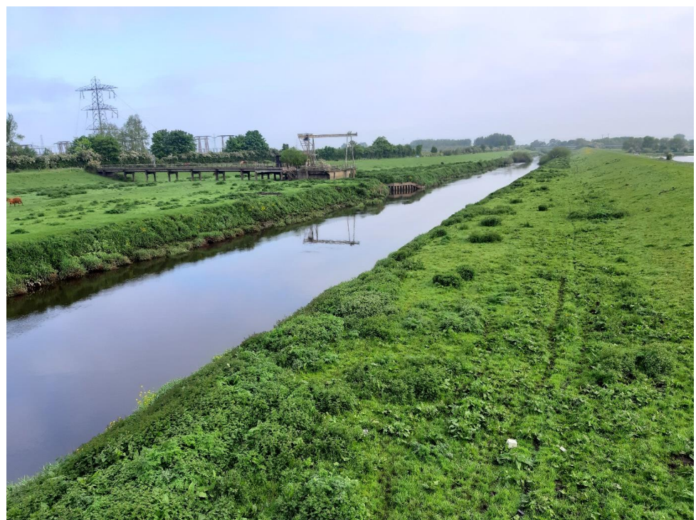
Figure 8. A straightened, deepened, and embanked reach of the lower River Don. Photograph: DCRT 2021.
