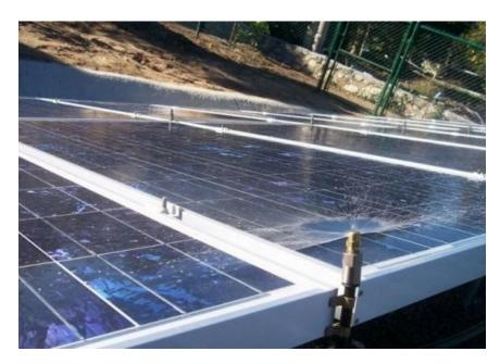
consumed for cleaning [44]. Figure 3 demonstrates the heliotex method of cleaning. This system is not suitable for all situations [19].
