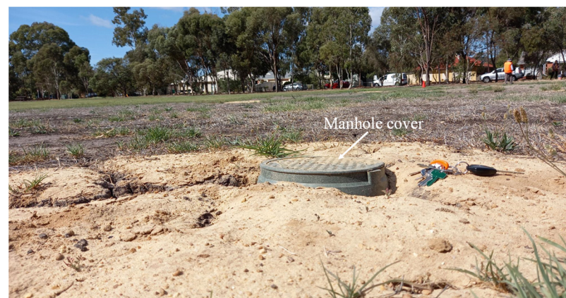
Figure 5. Surface cracks on the ground surface and settlement due to soil shrinkage around a manhole cover during dry season.
