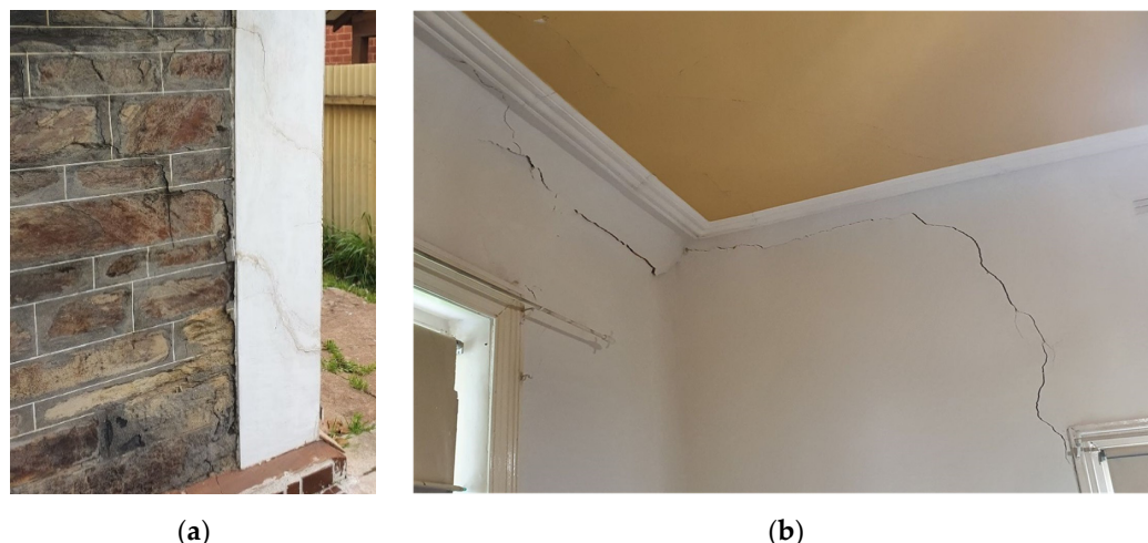
Figure 2. Damage to a building (a) due to edge heave; (b) due to centre heave.
