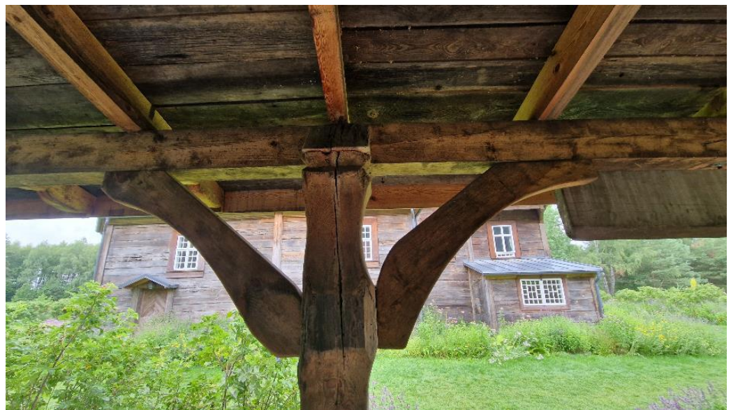
Figure 7. Carved structural elements of an overhang from historical wooden house in an open-air museum.
