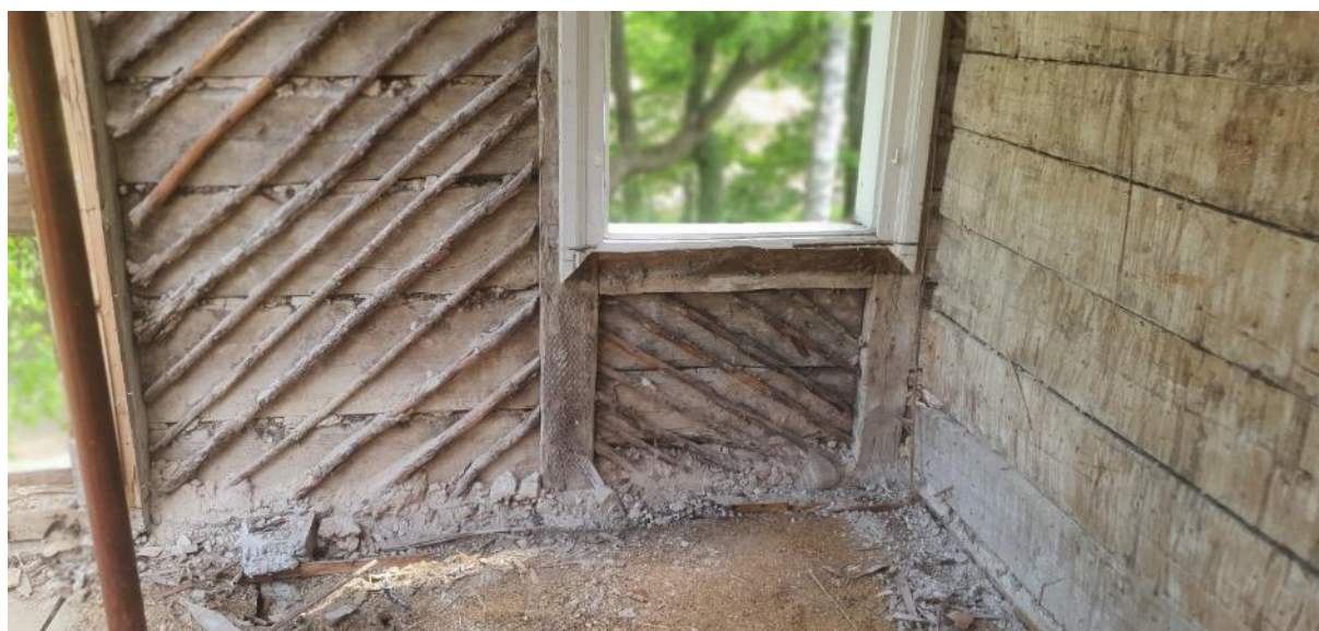
Figure 15. Historical thermal insulation installation method.
