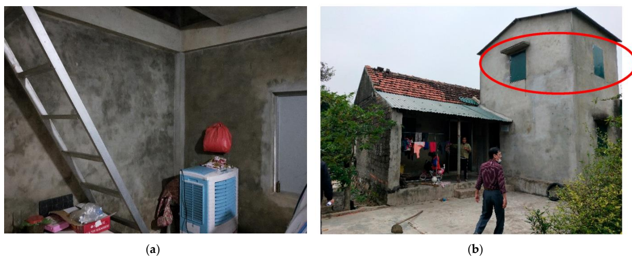
Figure 9. The project houses in Quang Binh province. (a) Permeable walls and narrow steps of ladder; (b) Side cover of the roof is missing.
