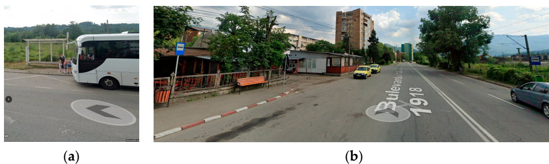
Figure 24. Route stations in Petrosani: (a) constructions of light metal structure; (b) stations without any facility.
