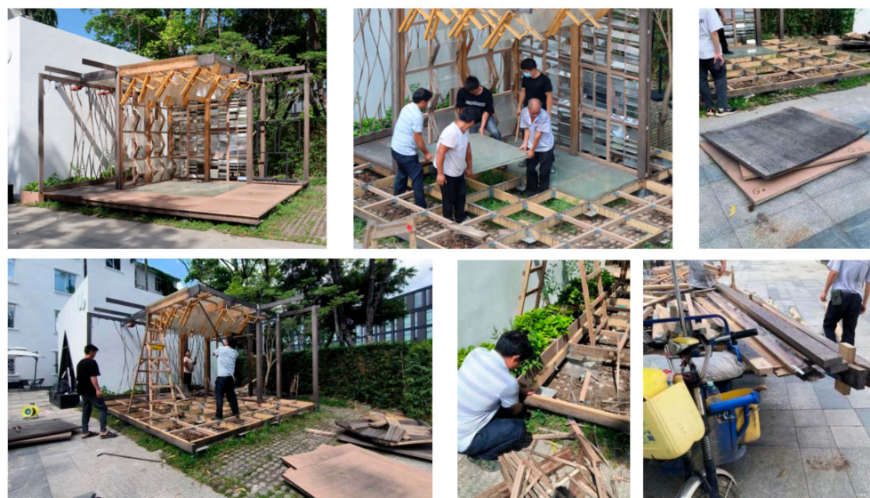
Figure 3. Disassembly process of Circular Pavilion ©REDO Design Corporation, Guangzhou, China.
