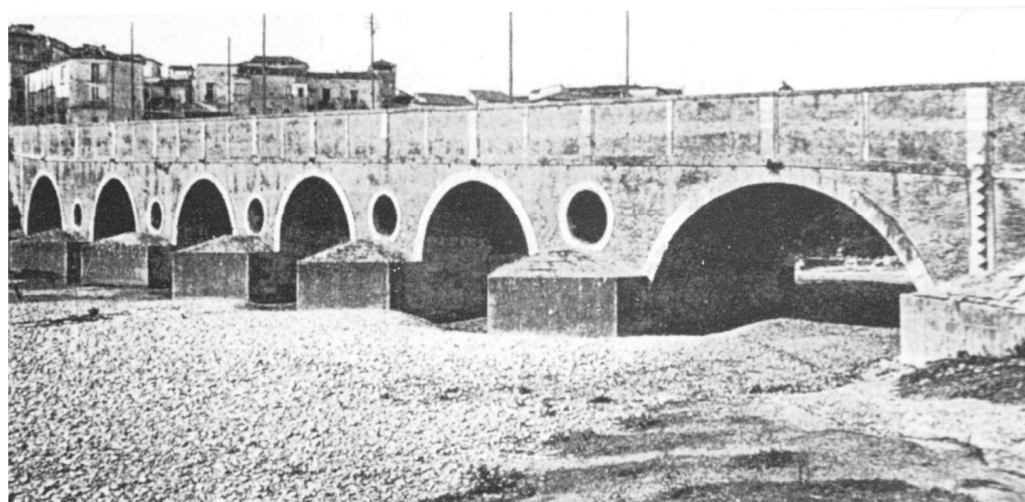
Figure 13. The bridge over the Calore in a photo taken before 1949, the year of its demolition following the high afflux effect exerted by the structure during the flood of the same year (source: [64]).
