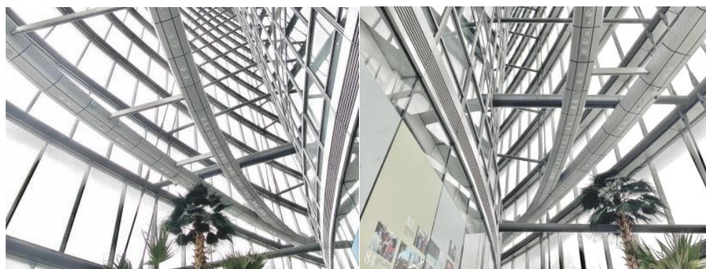
Figure 6. Actual scene photos of double-skin enclosure structure.
