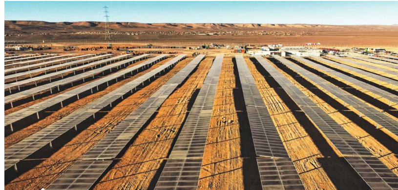
Figure 9. Rubi solar photovoltaic facility located in a desert landscape in Peru.
