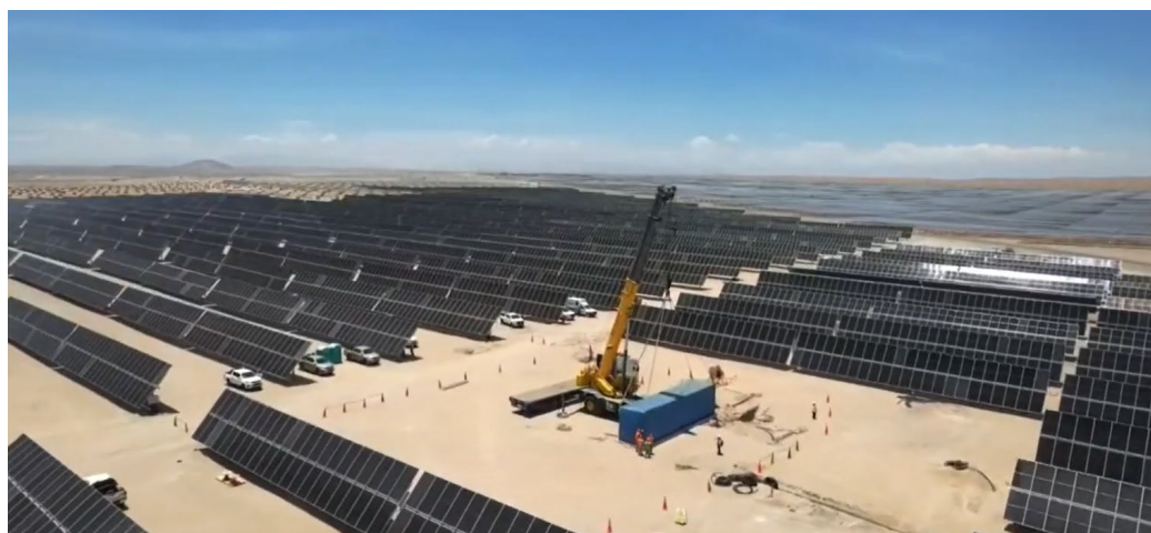
Figure 22. Landscape showing the San Martin solar photovoltaic facility under construction.
