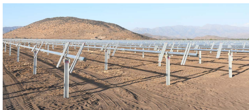
Figure 23. Landscape showing the Lupi solar photovoltaic facility under construction.
