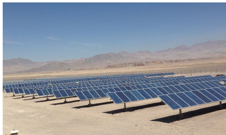
Figure 10. Landscape showing photovoltaic panels in the Repartición solar facility.
