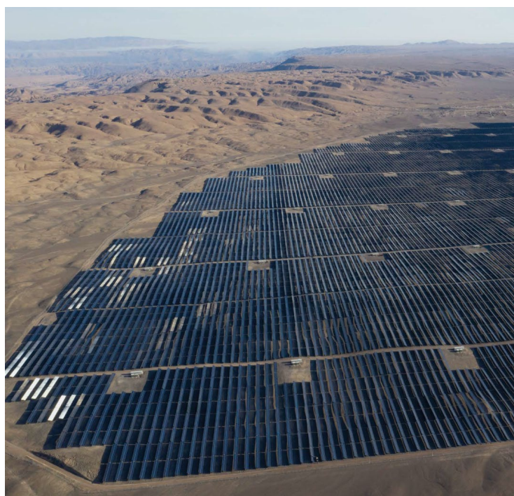
Figure 3. Rubi solar photovoltaic facility, located in a desert landscape in Peru.
