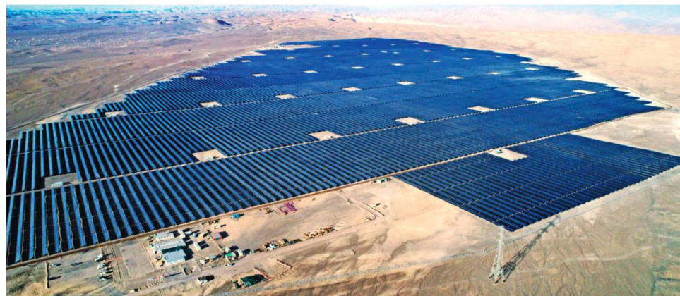
Figure 16. Landscape showing photovoltaic panels in the Rubi solar facility.
