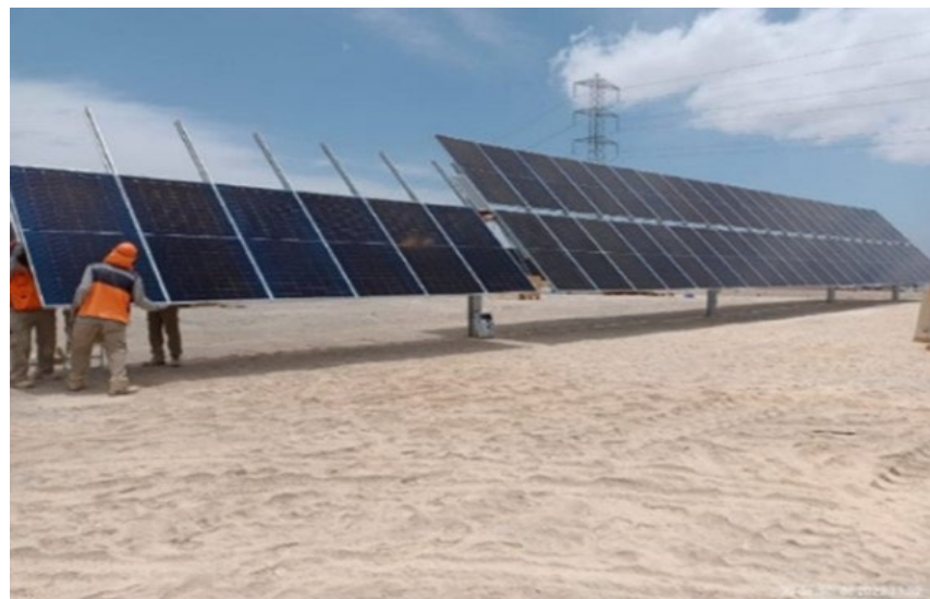
Figure 24. Landscape showing the Matarani solar photovoltaic facility under construction.
