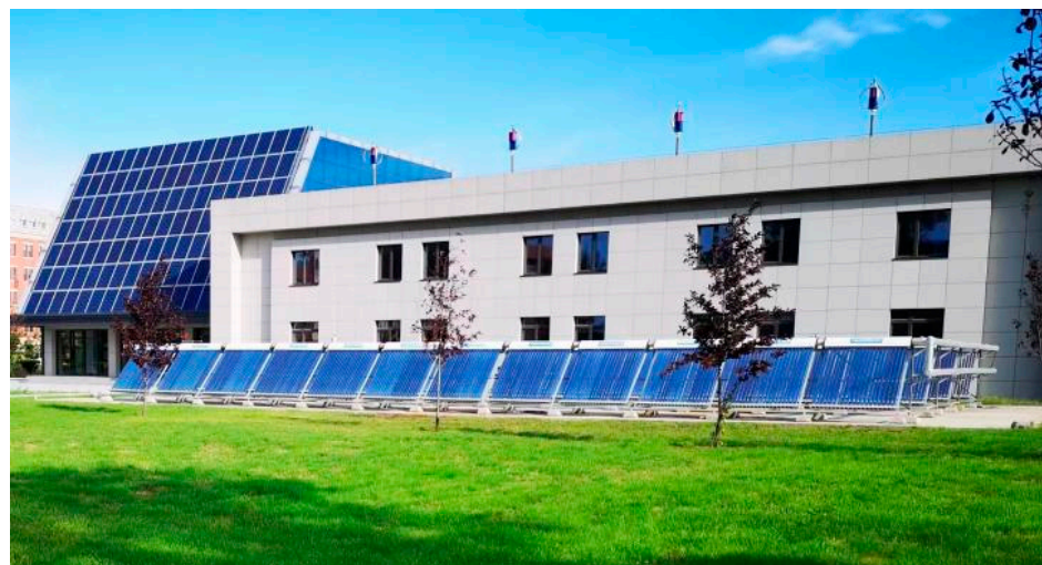
Figure 4. Building exterior view.
