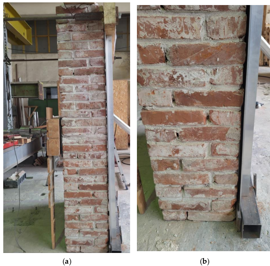
Figure 15. Imperfect adhesion between masonry support and aluminium alloy profiles; (a) Lateral View; (b) A detailed view of the imperfect adhesion.
