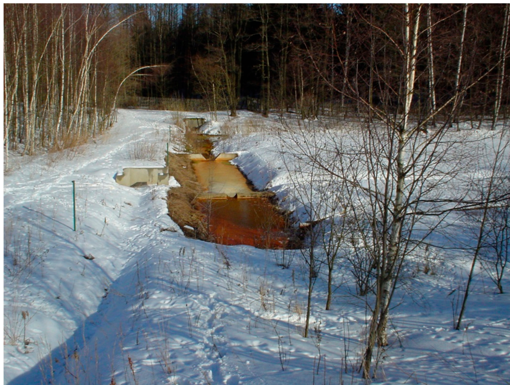
Figure 1. Hajek drainage channel.
