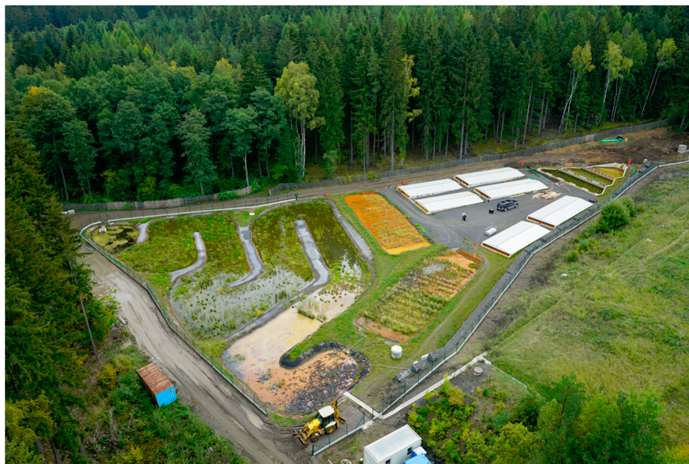
Figure 4. Wetland + installation in Hajek—aerial view.
