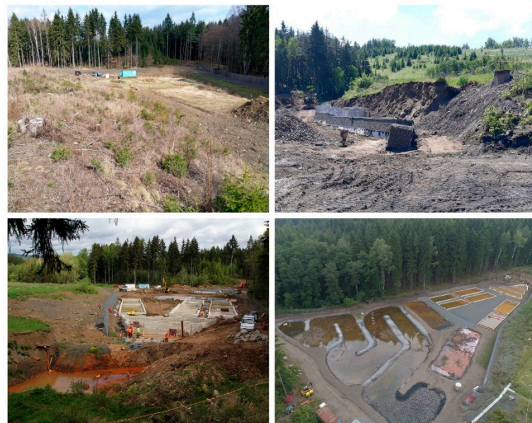
Figure 3. Wetland + installation in Hajek.
